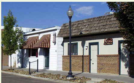
▲ Businesses along Lake Ave. between 1st & 2nd Streets are original structures.
