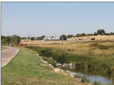
Grange Hall Creek at Margaret W. Carpenter Park & Open Space
