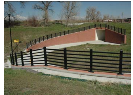
Underpass at 104th Avenue connects Grandview Ponds Open Space & Prairie Dog Habitat to Riverdale Open Space & Prairie Dog Habitat
