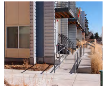
Housing for seniors and persons with disabilities located in close proximity to the transit station encourages an inclusive community.
