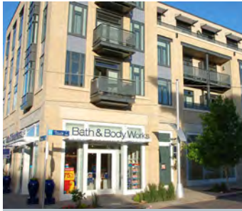
Storefront windows and architectural features in a mixed-use project create visual interest for pedestrians.
