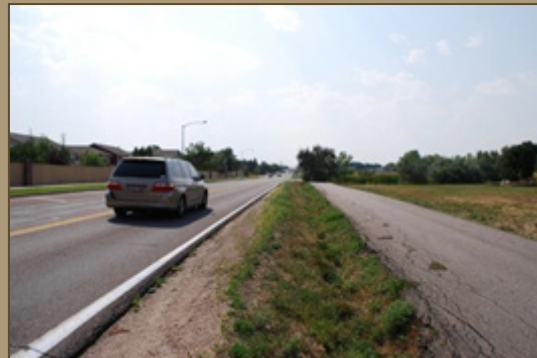
Shared bicycle/pedestrian path on north side of 112th Ave. can create conflicts for both types of users....
