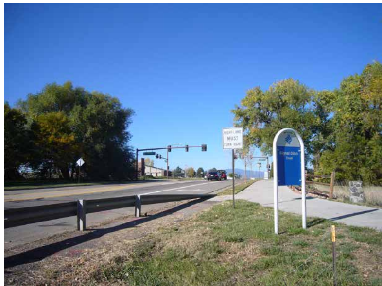
Signal Ditch Trail at 128th & Lafayette St.
