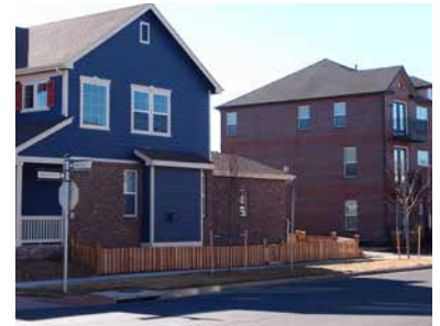
Transitioning densities from multifamily to single-family residential development ensure compatibility with surrounding neighborhoods
