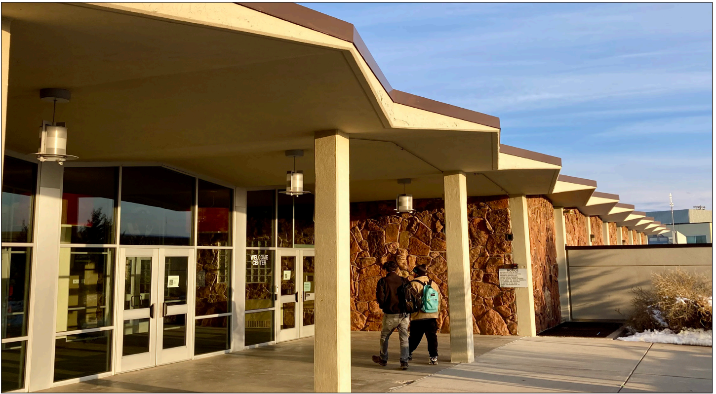
Students walking under an exuberant fan-like canopy at the Mapleton School District No. 1 building off of York Street.
