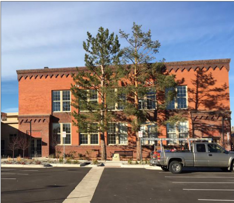
The historic Fruitdale School in Wheatridge that used tax credits in support of conversion to 16 apartments. Source: History Colorado
