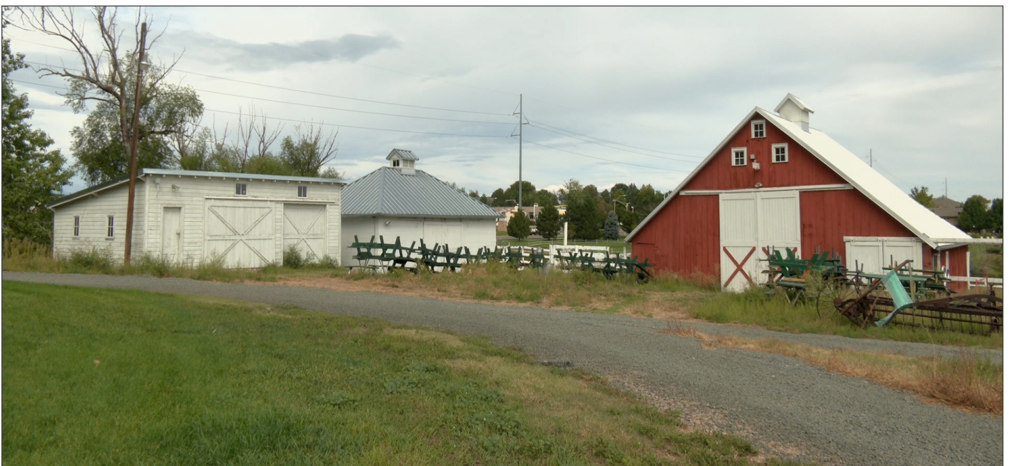
A view from the interior yard of the Lambertson Lakes Homestead property owned by the city of Thornton.
