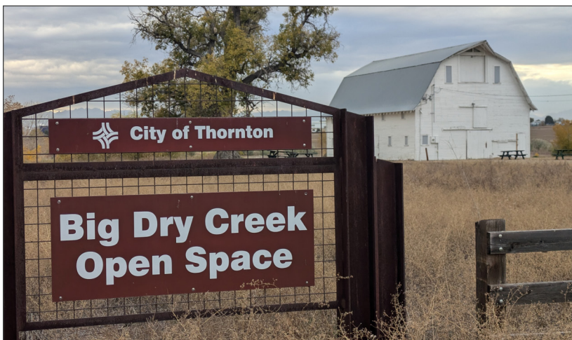
The Reitzenstein Barn, Thornton’s only locally listed historic landmark.
