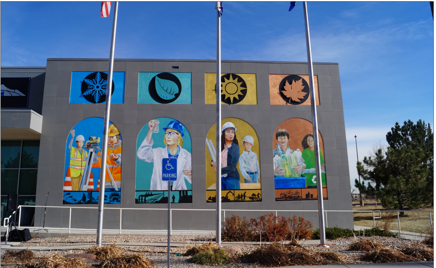
A mural on the western side of the Infrastructure Maintenance Center.
