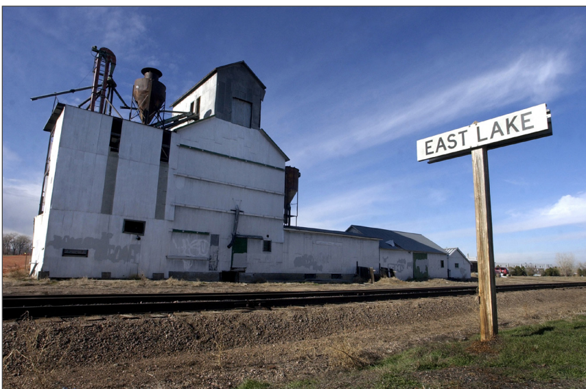
A side view of the Eastlake grain elevator, just before construction started on the Eastlake N Line Station.
