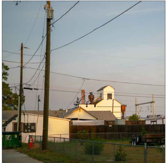
A view from an Eastlake residential alley with the Eastlake grain elevator in the background.
